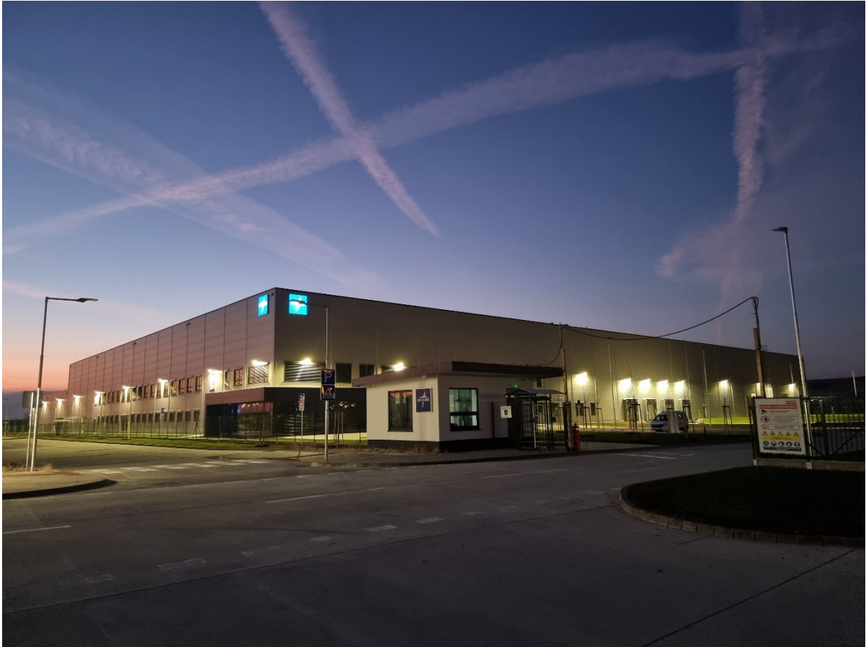
MEDLINE production and warehouse hall, Malé Bělčice
