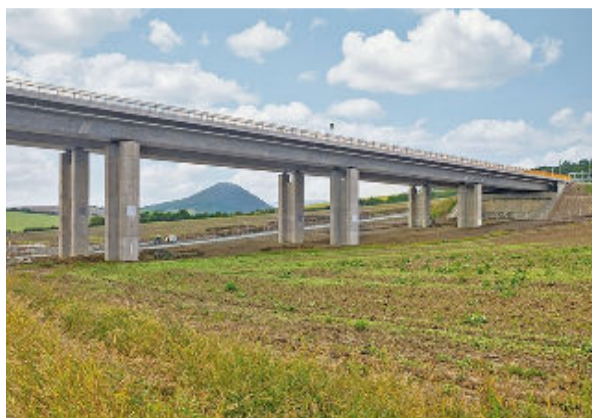
Most na R4 v km 1,350 (SO 201-00)
