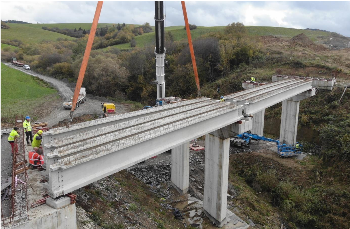
Bridge over the future R3, Nižná – Tvrdošín
