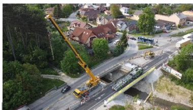
Bridge girders on the Road E75 for the bridge near the village Radoľa
