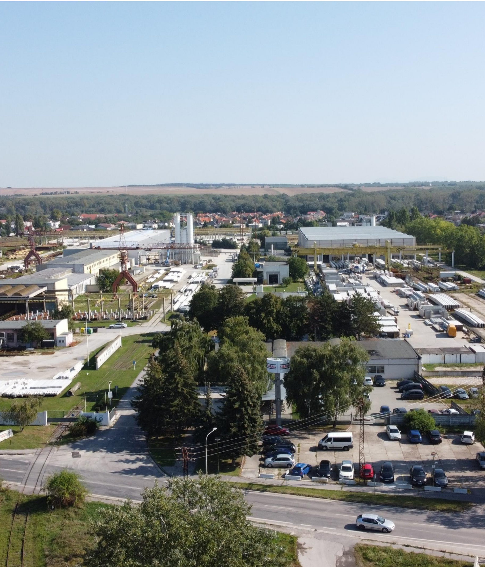
Plant STRABAG Sered, production, transport and assembly of precast concrete
