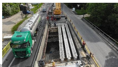
Bridge girders on the Road E75 for the bridge near the village Radoľa
