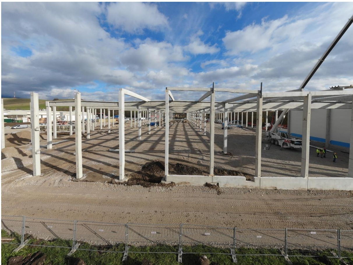
Assembly of the prefabricated hall skeleton for HOVAL, Istebné
