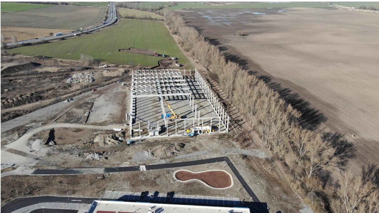
Installation of prefabricated reinforced concrete skeleton for the company VGP, Zvolen
