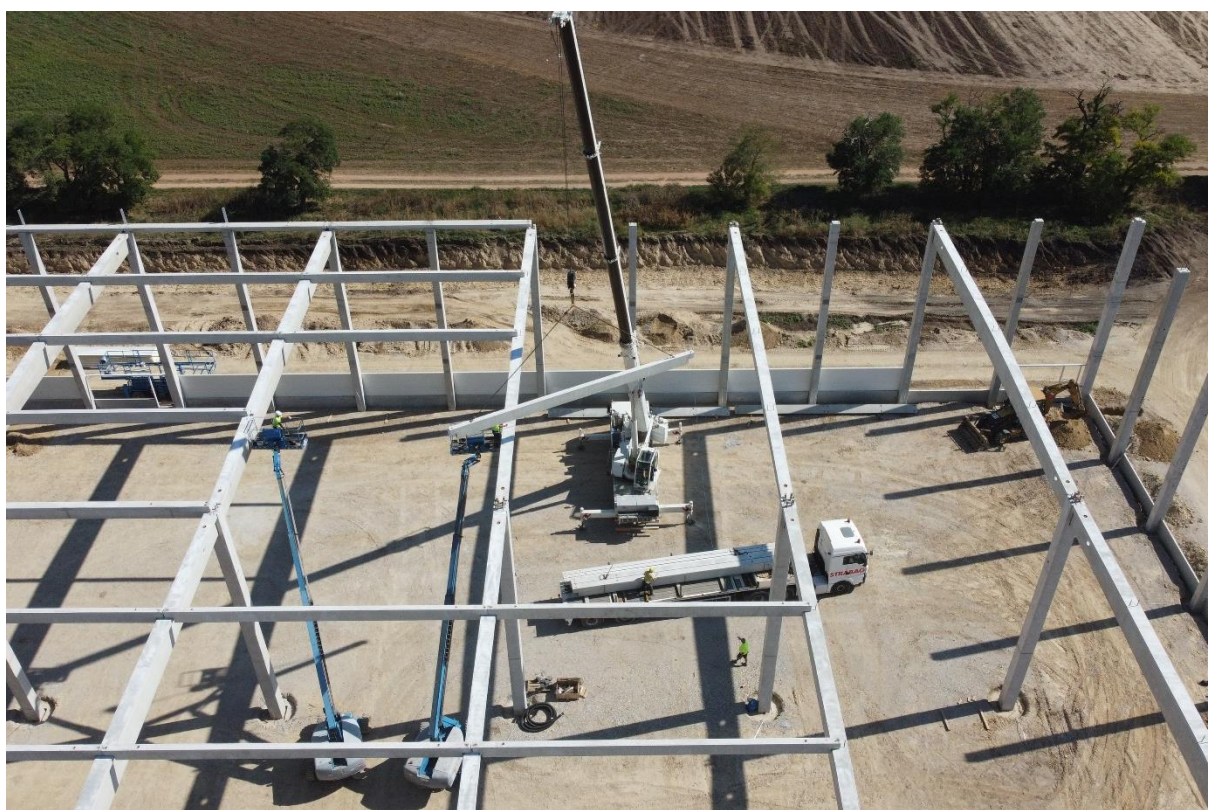
Installation of prefabricated reinforced concrete skeleton for the company CTPark, Voderady
