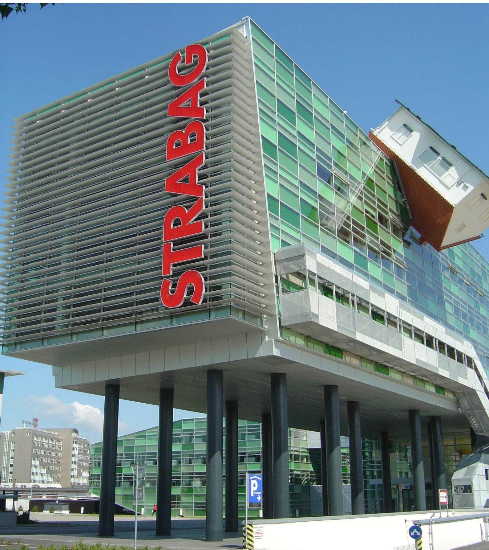
Headquarters Bratislava, seat of the company
