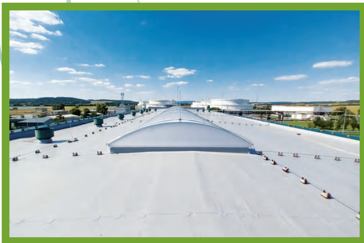
Photo: Reconstructed roof of the ADRIA Workshop at PS4 Tupá.
