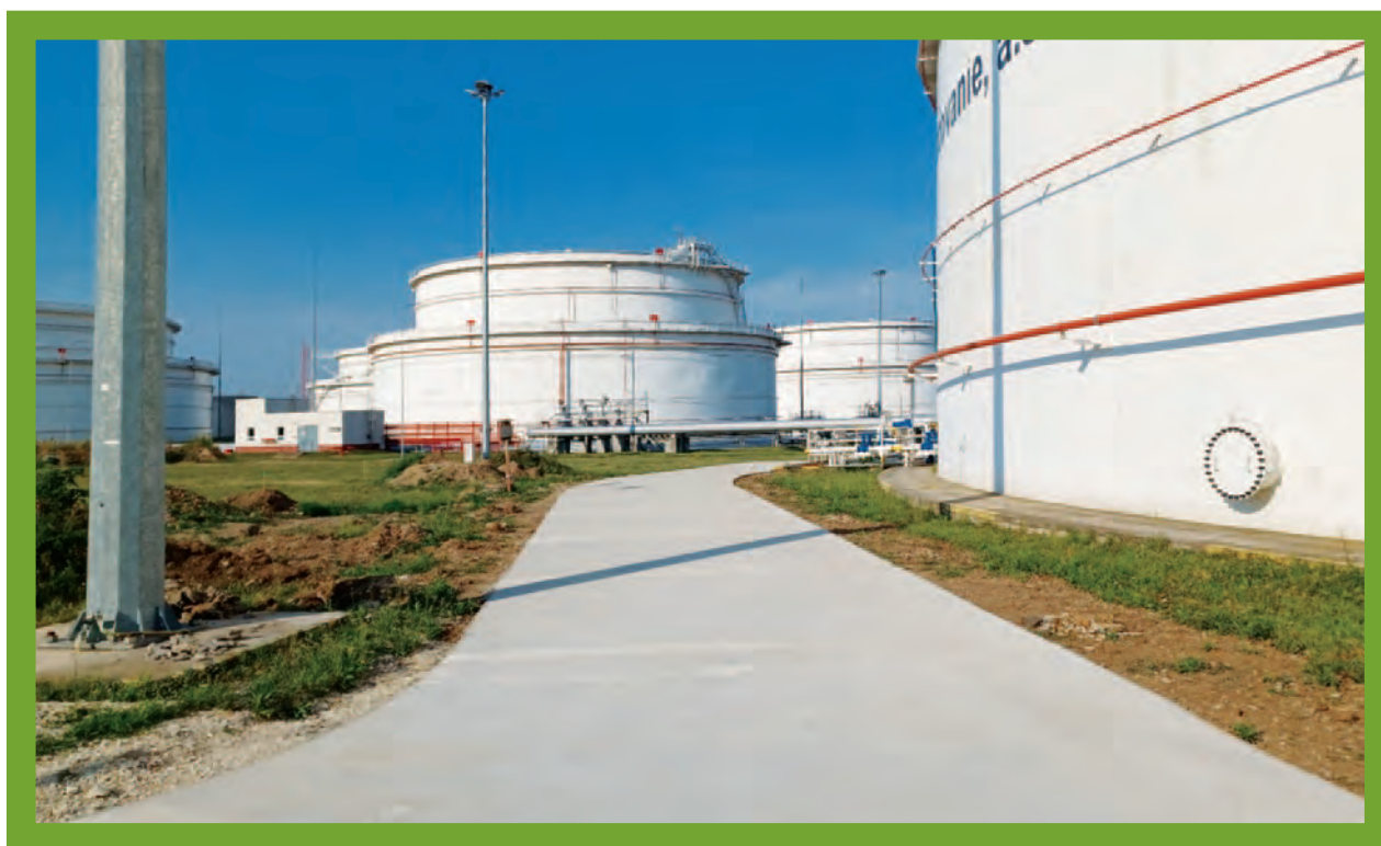
Photo: New road to the side sludge tanks of the large-capacity tanks at PS4 Tupá.
