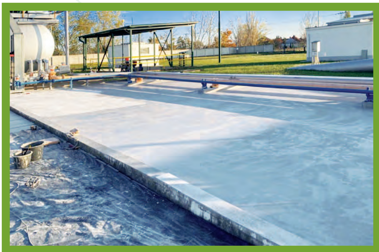
Photo: Reconstructed decanting areas at PS5 Bučany.
