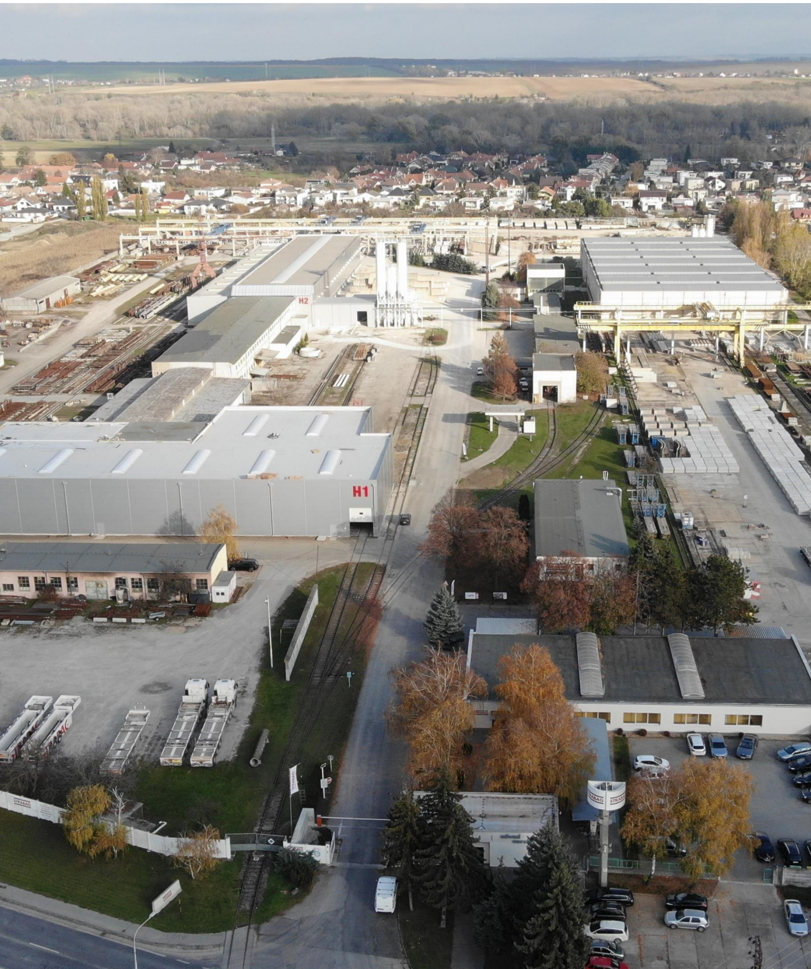
Plant STRABAG Sered, production, transport and assembly of precast concrete
