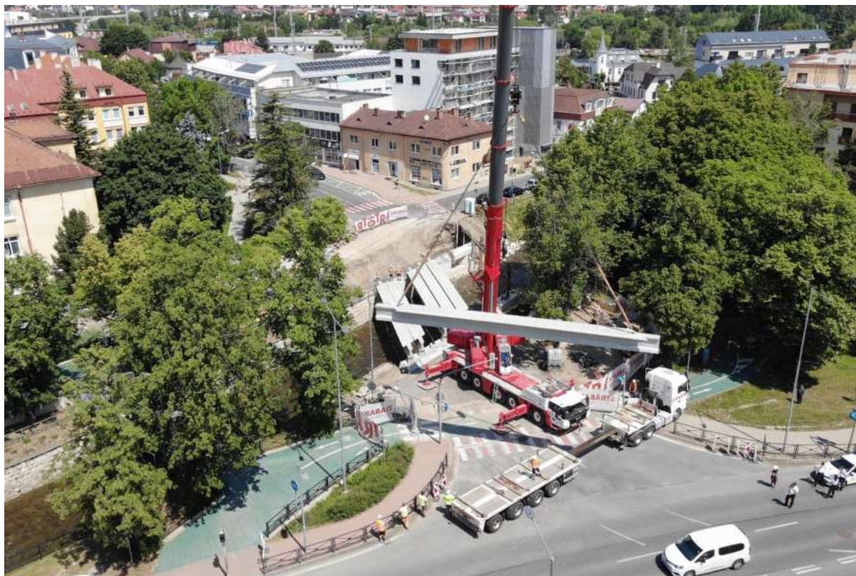
Bridge Construction, Poprad
