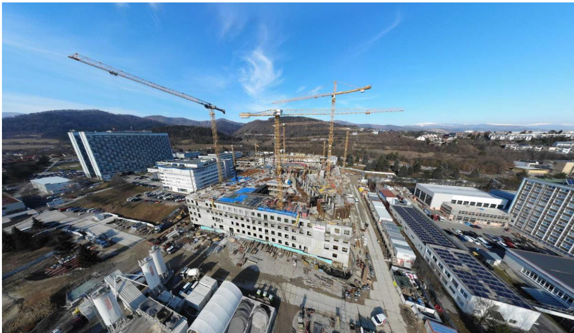
Construction of the F. D. Roosevelt University Hospital, Banská Bystrica
