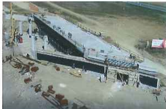
Most na R2 nad III/2640 v km 19.555
