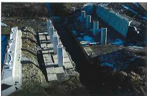
Most na R2 v km 11,450
