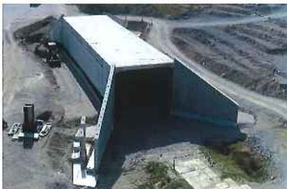
Most na R2 nad PC v km 9,000
