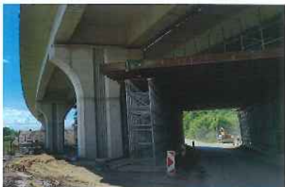
Most na R2 nad III/2664 v km 15.400
