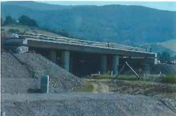
Most na R2 nad III/2632 v km 10.500
