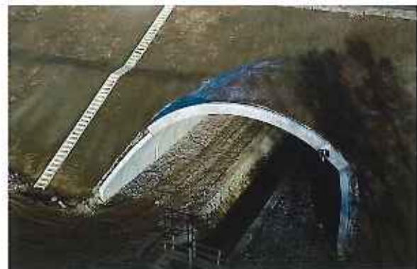
Most na R2 nad potokom Udorinka v km 18.450
